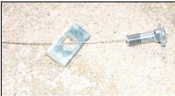
Hidden Hitch provided “feeder” lines to help fish the new bolts to their locations in the frame rail.
